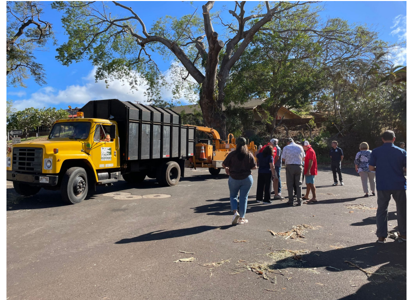
Debris clean up at Lāhaināluna High
